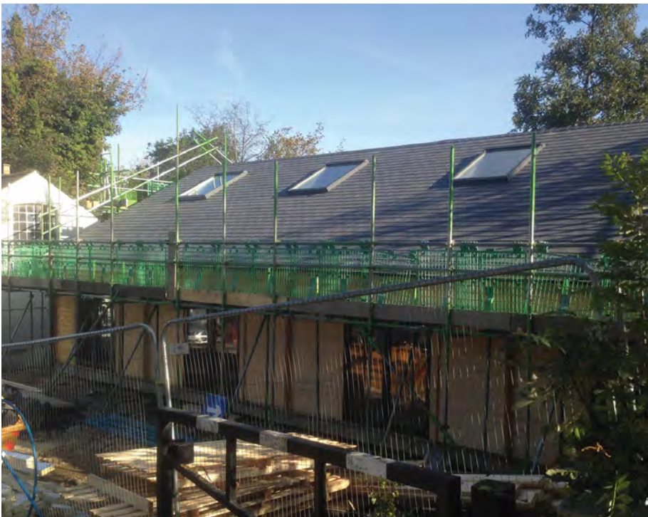
Building Under Construction (a)
