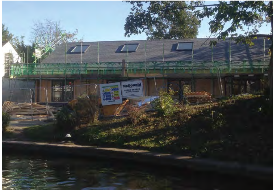
Building Under Construction (b)
