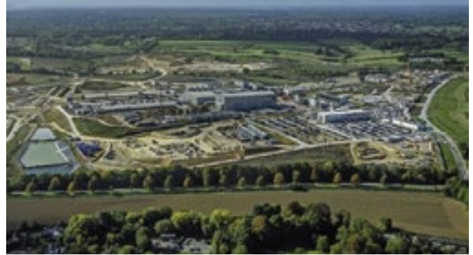
Viaduct crossing the North Orbital Road
