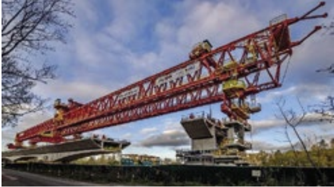
Viaduct crossing the North Orbital Road
