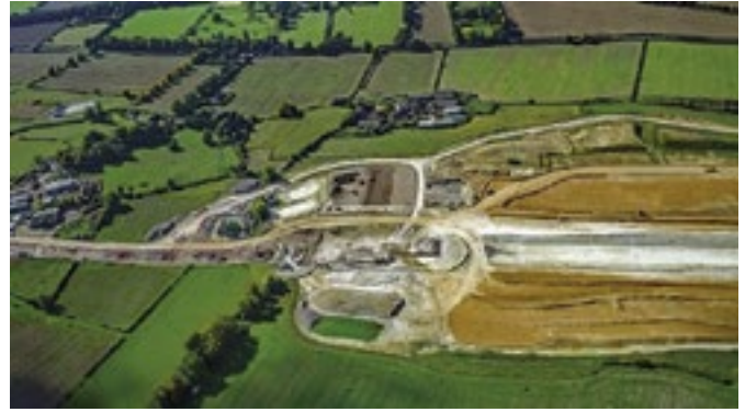
Wendover Dean viaduct looking west towards the A413
