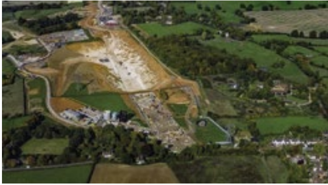
The Chiltern Tunnel north portal north of Frith Hill, South Heath
