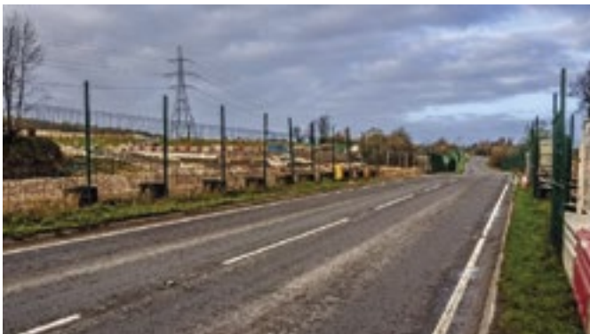
Small Dean viaduct crossing the A413 south of Wendover
