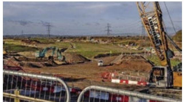
The Wendover green tunnel looking north from Ellesborough road diversion
