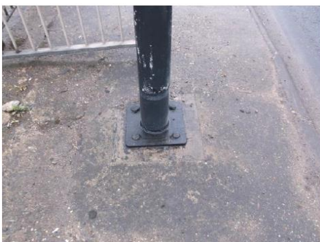
Beacon post flange base fixing on central reserve
