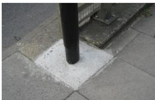
Beacon pole in footway; southbound carriageway
