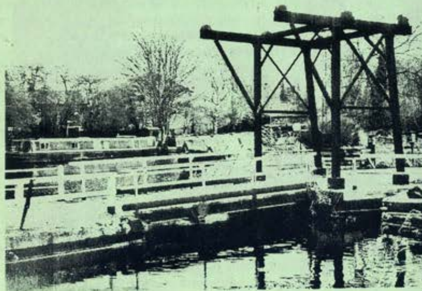
River Chess - Chess Basin Lifting Bridge, Rickmansworth
